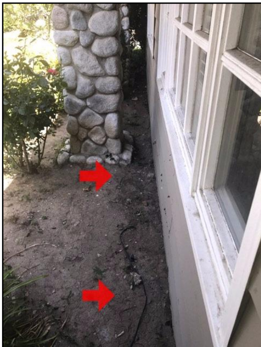
31. Improper slope or drainage
