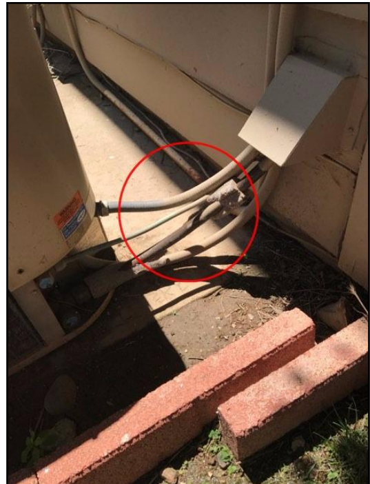
49. Insulation - missing
