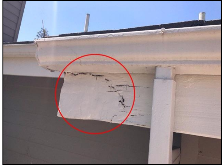
6. Rot or insect damage
