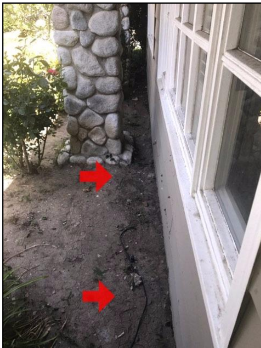
120. Improper slope or drainage
