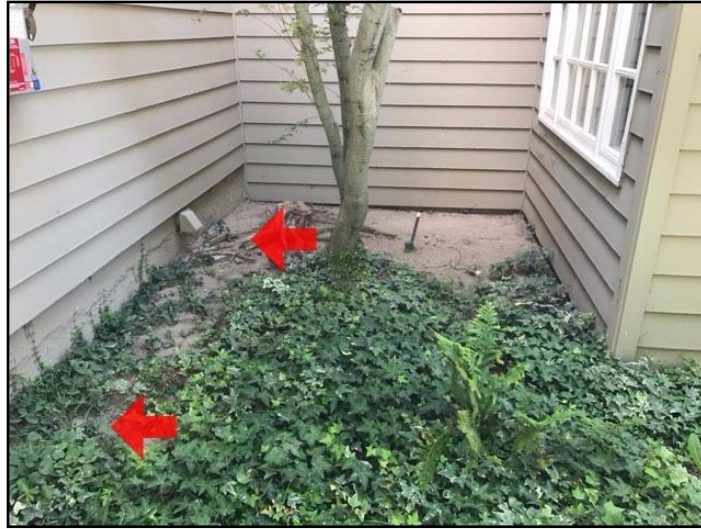
122. Improper slope or drainage
