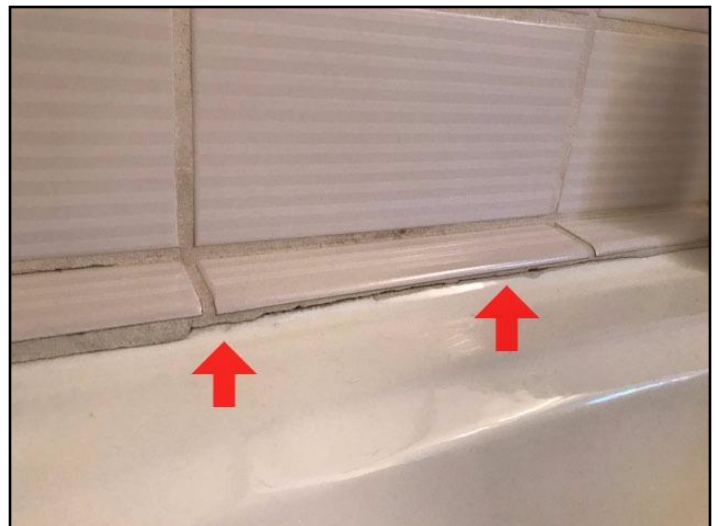
147. Grout loose, missing or deteriorated
