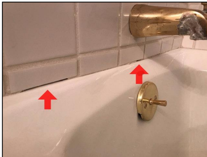
148. Grout loose, missing or deteriorated
