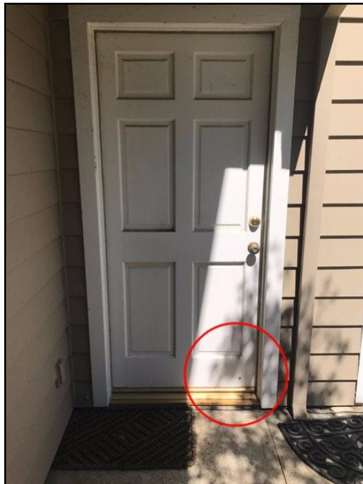
23. Rot or insect damage
