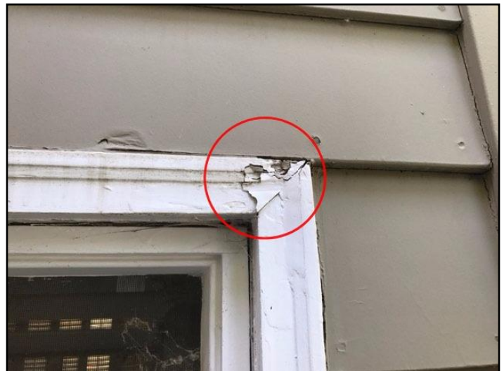
110. Rot or insect damage
