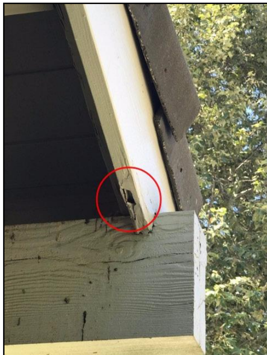
3. Rot or insect damage
