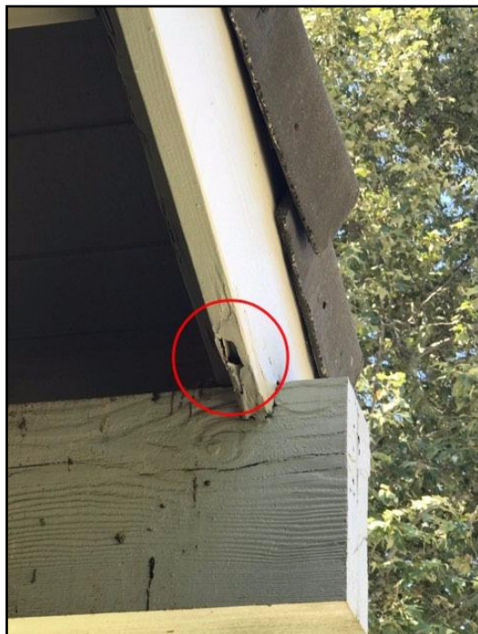
92. Rot or insect damage
