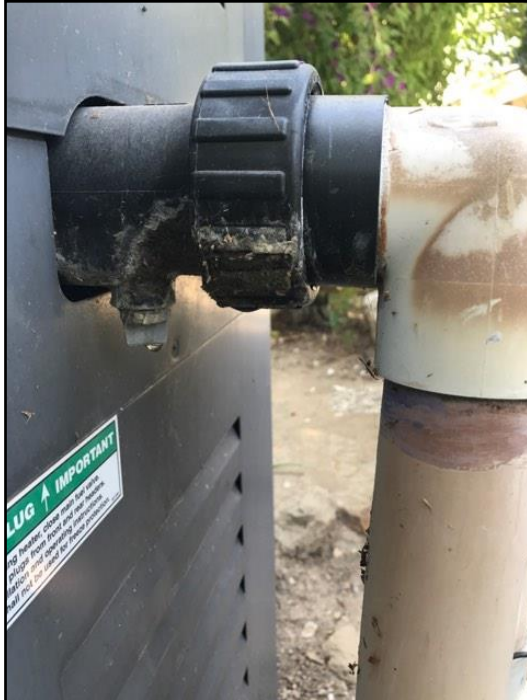
153. Pump leaking
