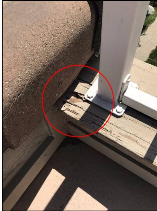
28. Rot or insect damage
