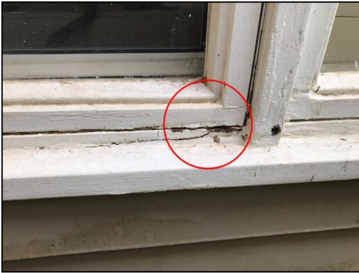
107. Rot or insect damage
