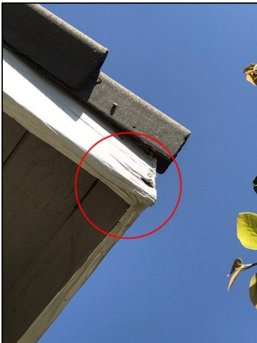
7. Rot or insect damage
