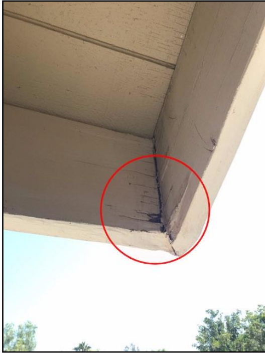
9. Rot or insect damage
