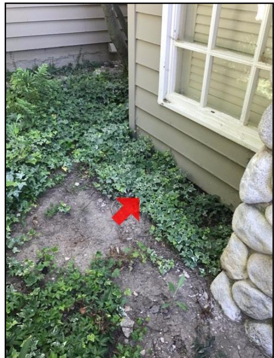
121. Improper slope or drainage
