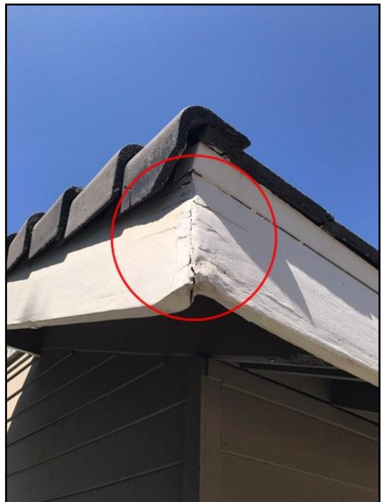
101. Rot or insect damage
