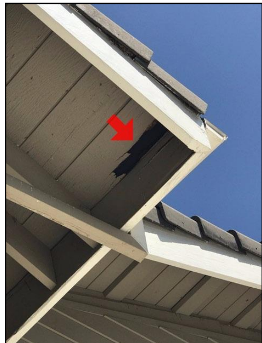
93. Rot or insect damage
