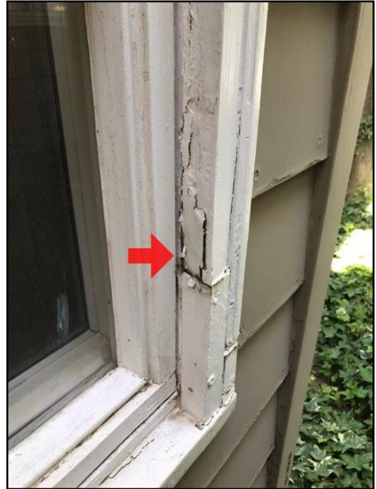
19. Rot or insect damage
