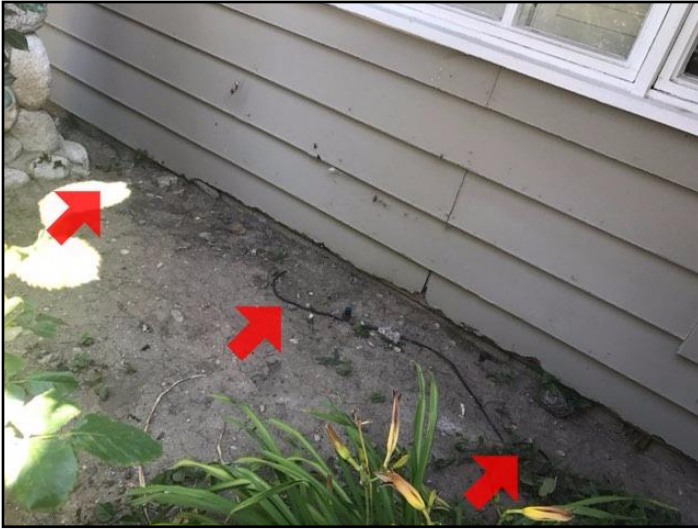
29. Improper slope or drainage
