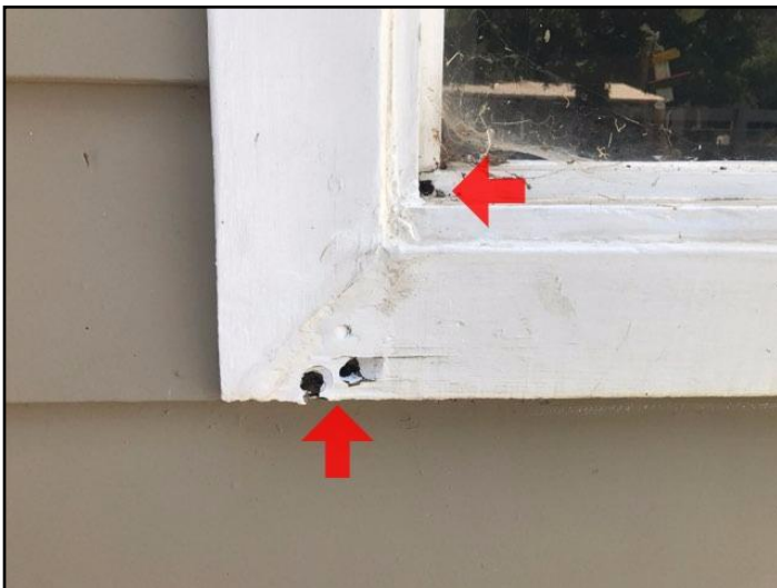
109. Rot or insect damage
