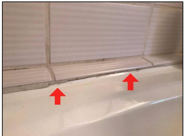
54. Grout loose, missing or deteriorated
