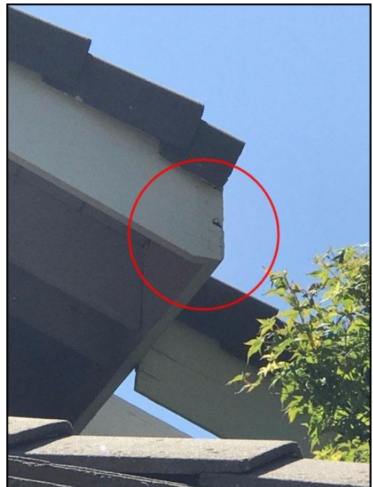
97. Rot or insect damage
