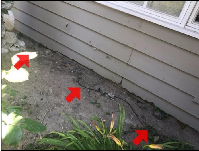
118. Improper slope or drainage
