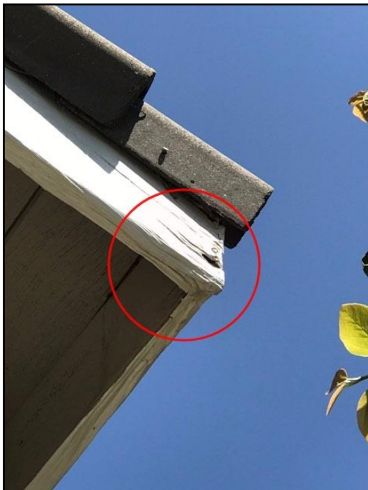
96. Rot or insect damage
