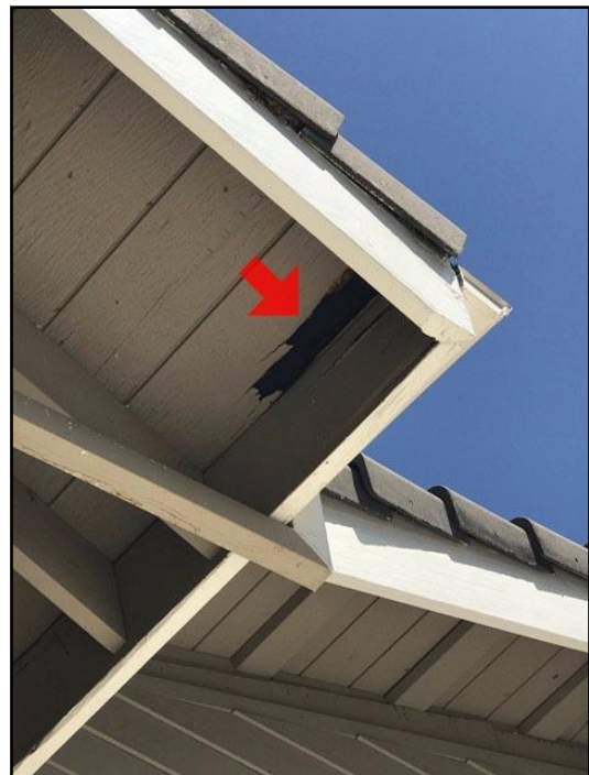
4. Rot or insect damage
