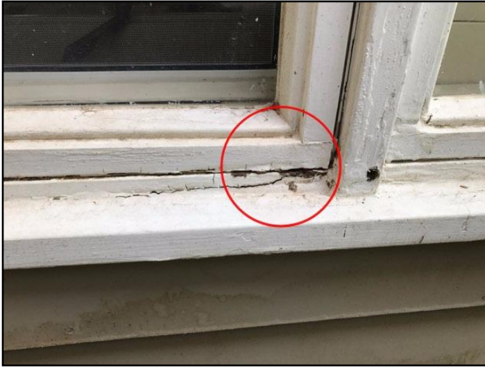
18. Rot or insect damage
