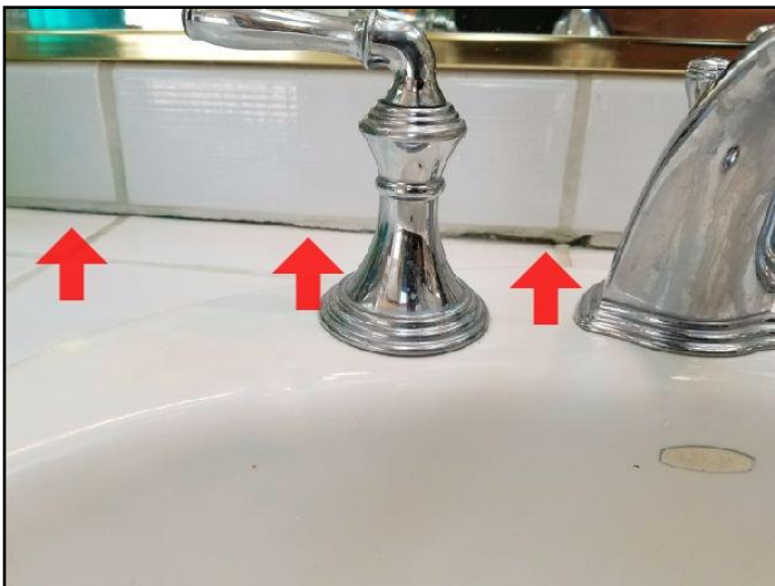
185. Grout loose or missing
