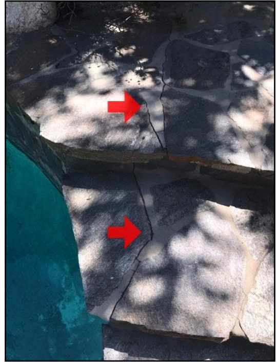
57. Surrounding deck/concrete cracked
