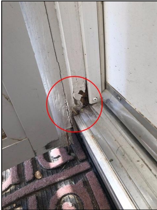
114. Rot or insect damage
