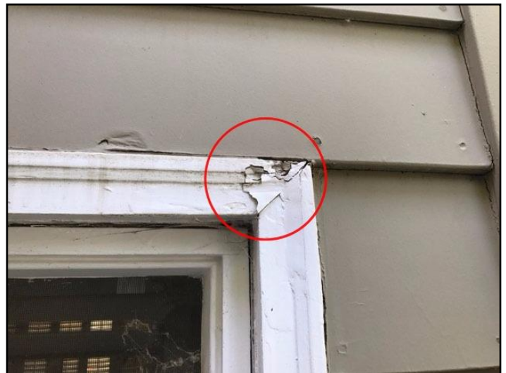
21. Rot or insect damage
