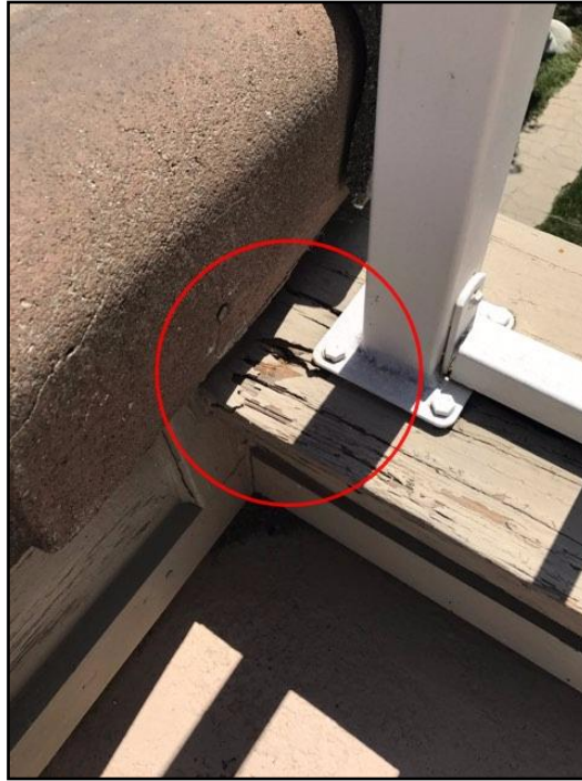
117. Rot or insect damage
