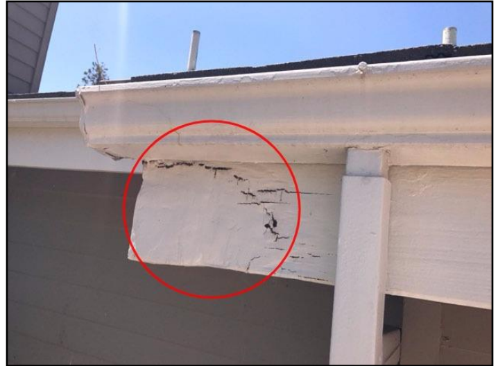
95. Rot or insect damage
