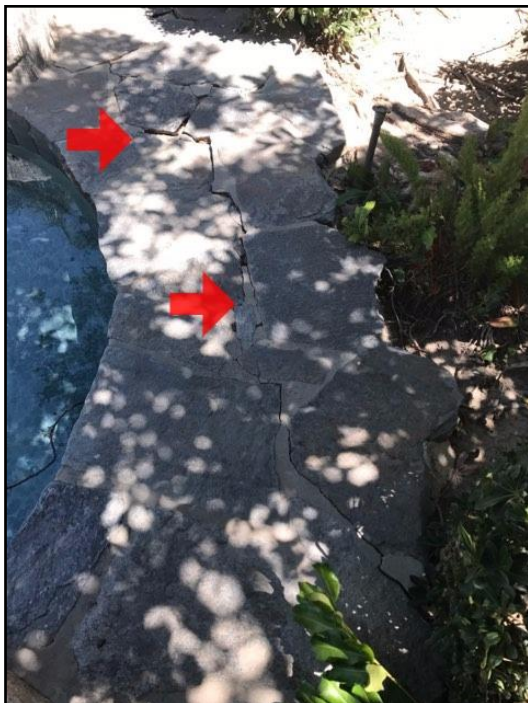
58. Surrounding deck/concrete cracked
