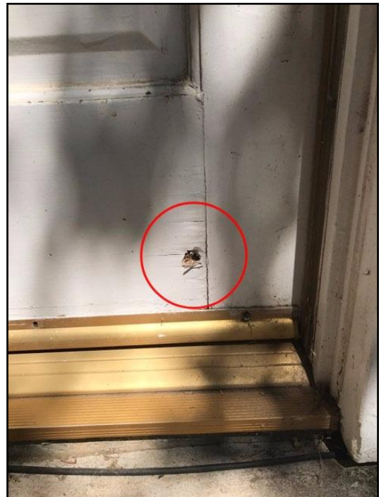
24. Rot or insect damage
