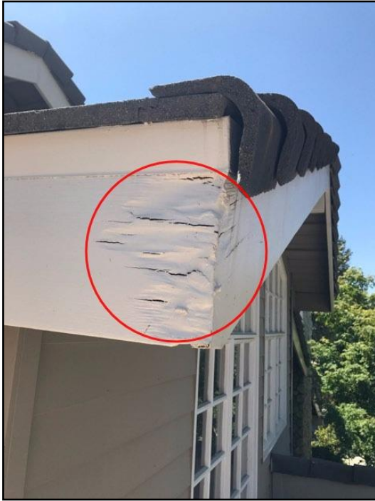
5. Rot or insect damage
