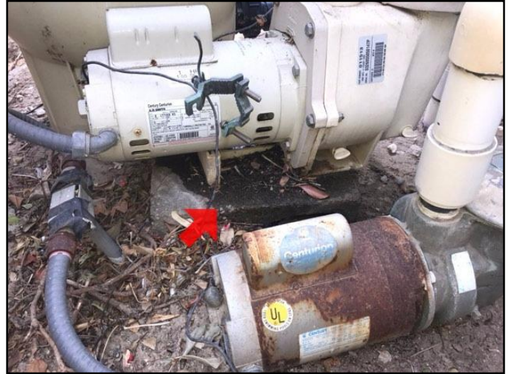
154. Pump leaking
