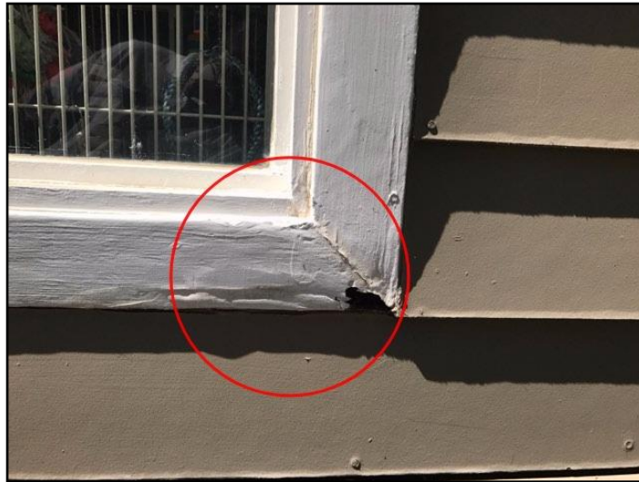
22. Rot or insect damage
