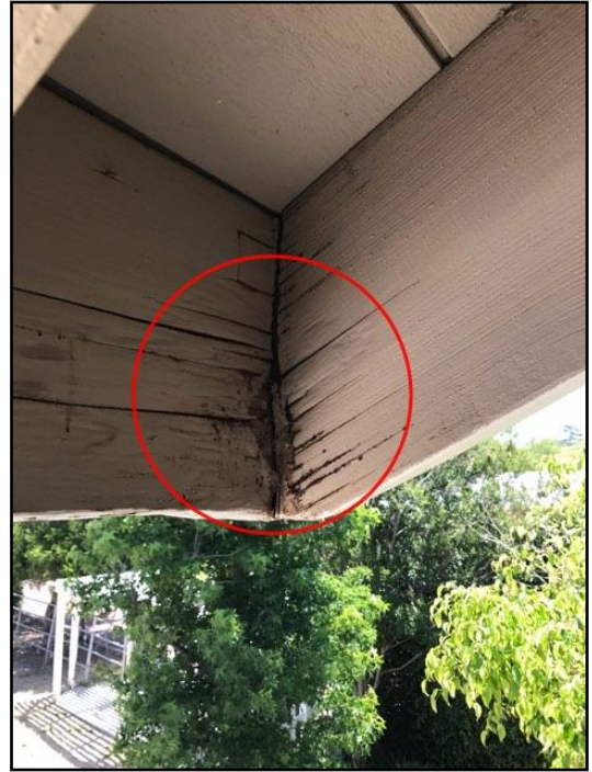
10. Rot or insect damage
