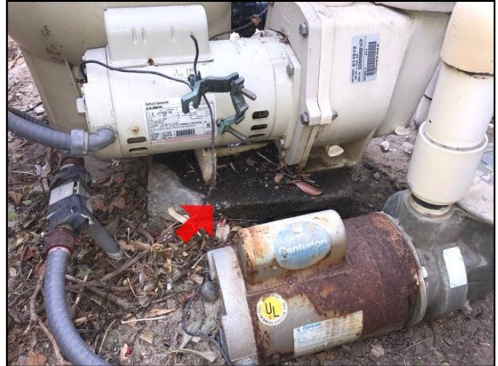
61. Pump leaking
