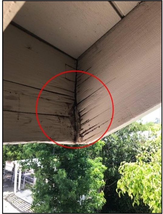
99. Rot or insect damage
