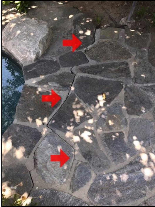
149. Surrounding deck/concrete cracked
