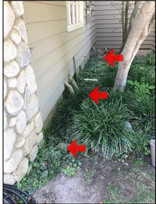
119. Improper slope or drainage
