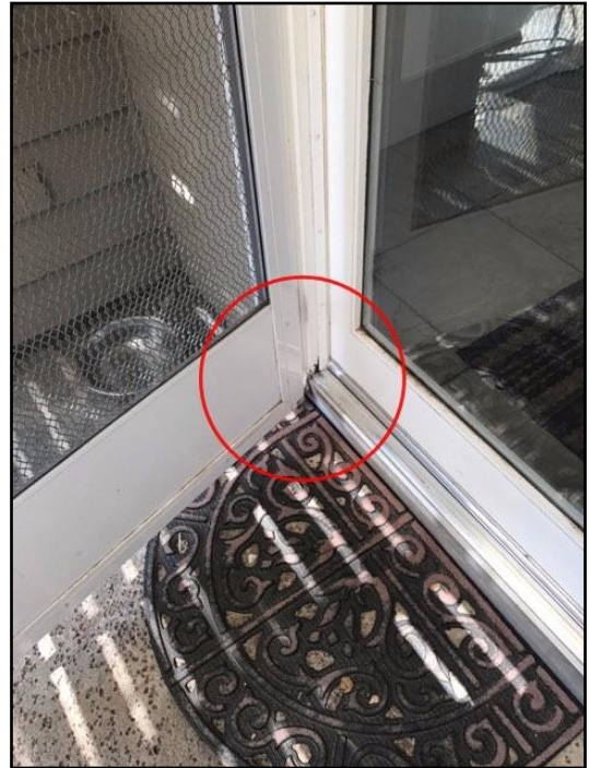
26. Rot or insect damage
