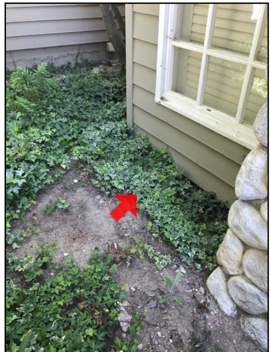
32. Improper slope or drainage
