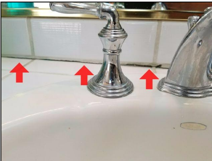
83. Grout loose or missing
