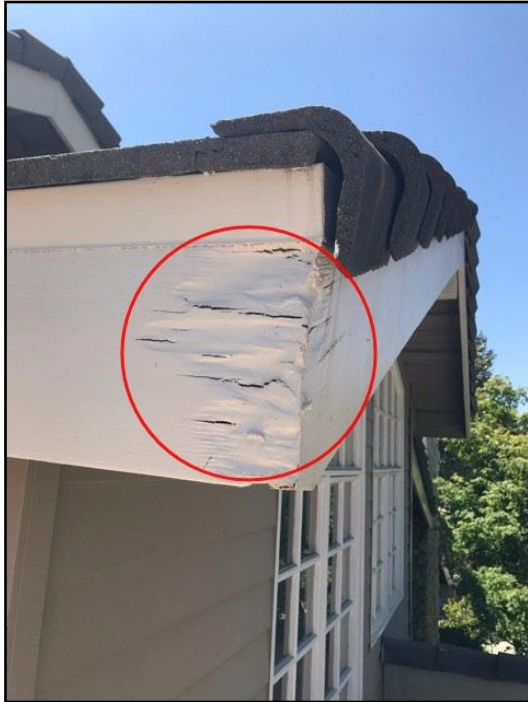
94. Rot or insect damage
