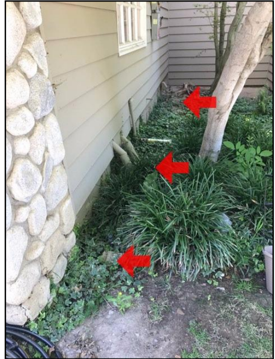
30. Improper slope or drainage
