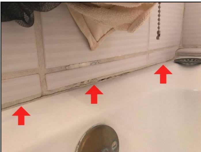
53. Grout loose, missing or deteriorated
