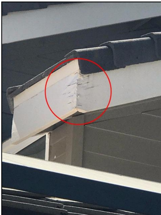
11. Rot or insect damage
