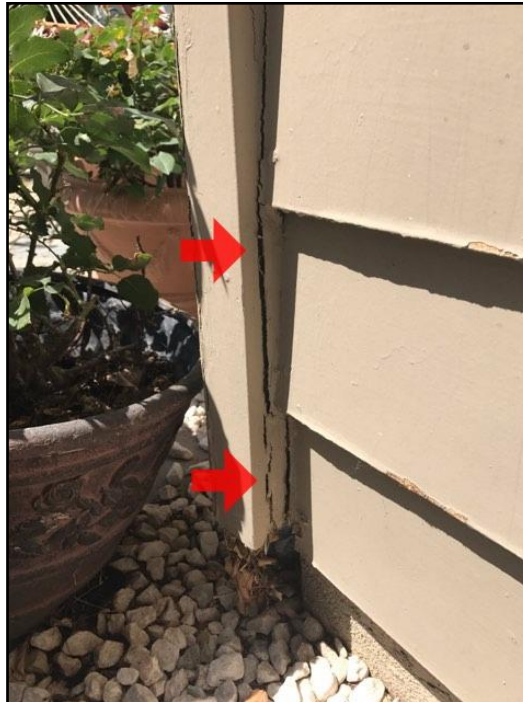
102. Rot or insect damage
