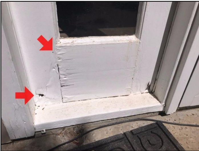
16. Rot or insect damage
