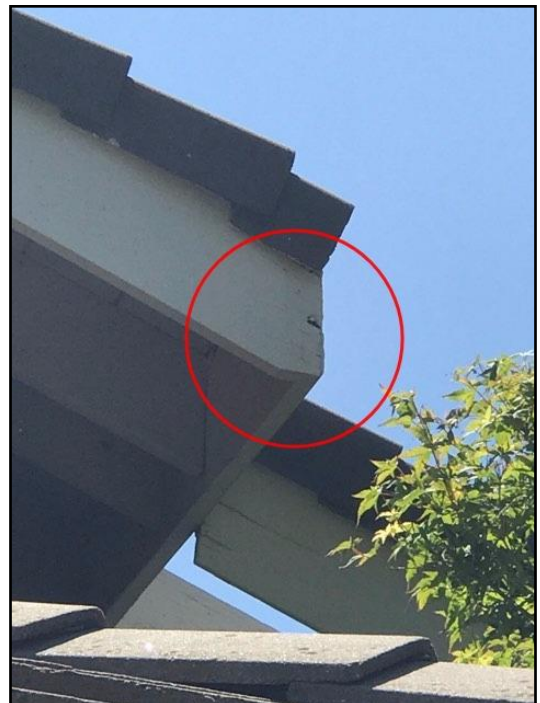
8. Rot or insect damage
