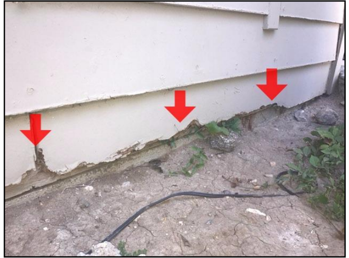
104. Rot or insect damage
