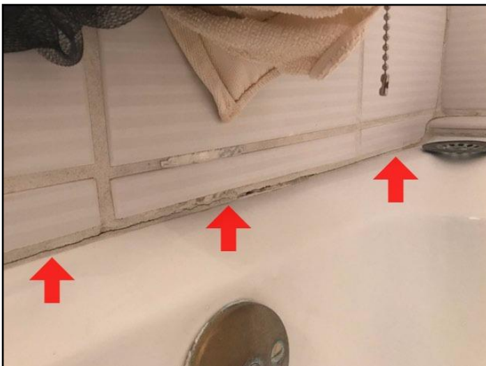
146. Grout loose, missing or deteriorated
