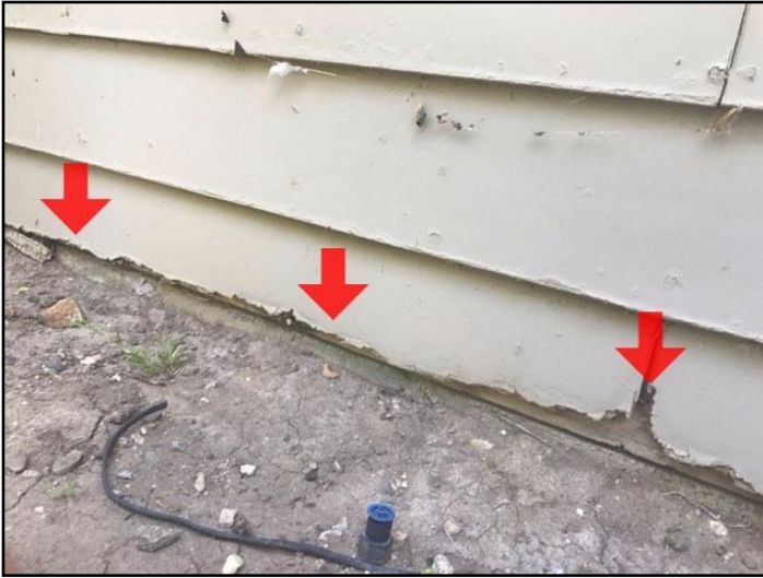
14. Rot or insect damage
