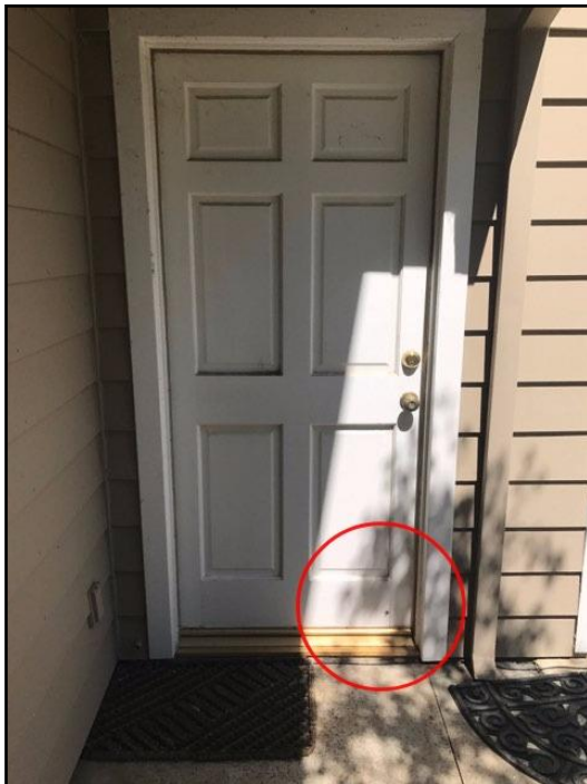
112. Rot or insect damage
