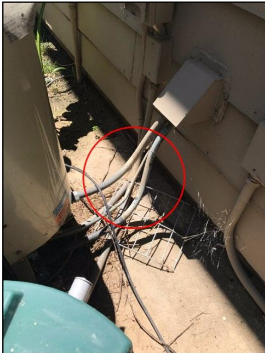
140. Insulation - missing
