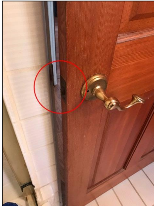
184. Does not latch properly
