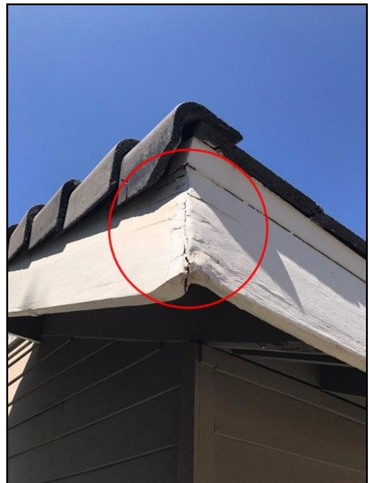
12. Rot or insect damage
