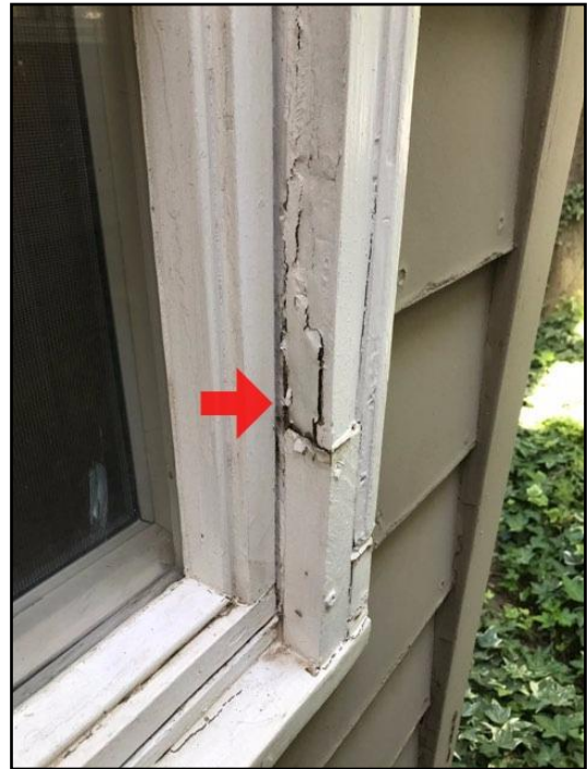
108. Rot or insect damage
