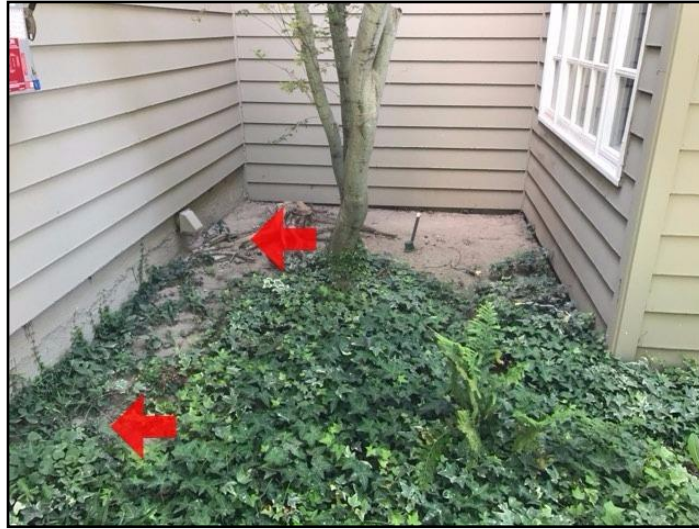
33. Improper slope or drainage
