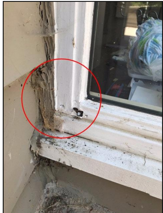
17. Rot or insect damage
